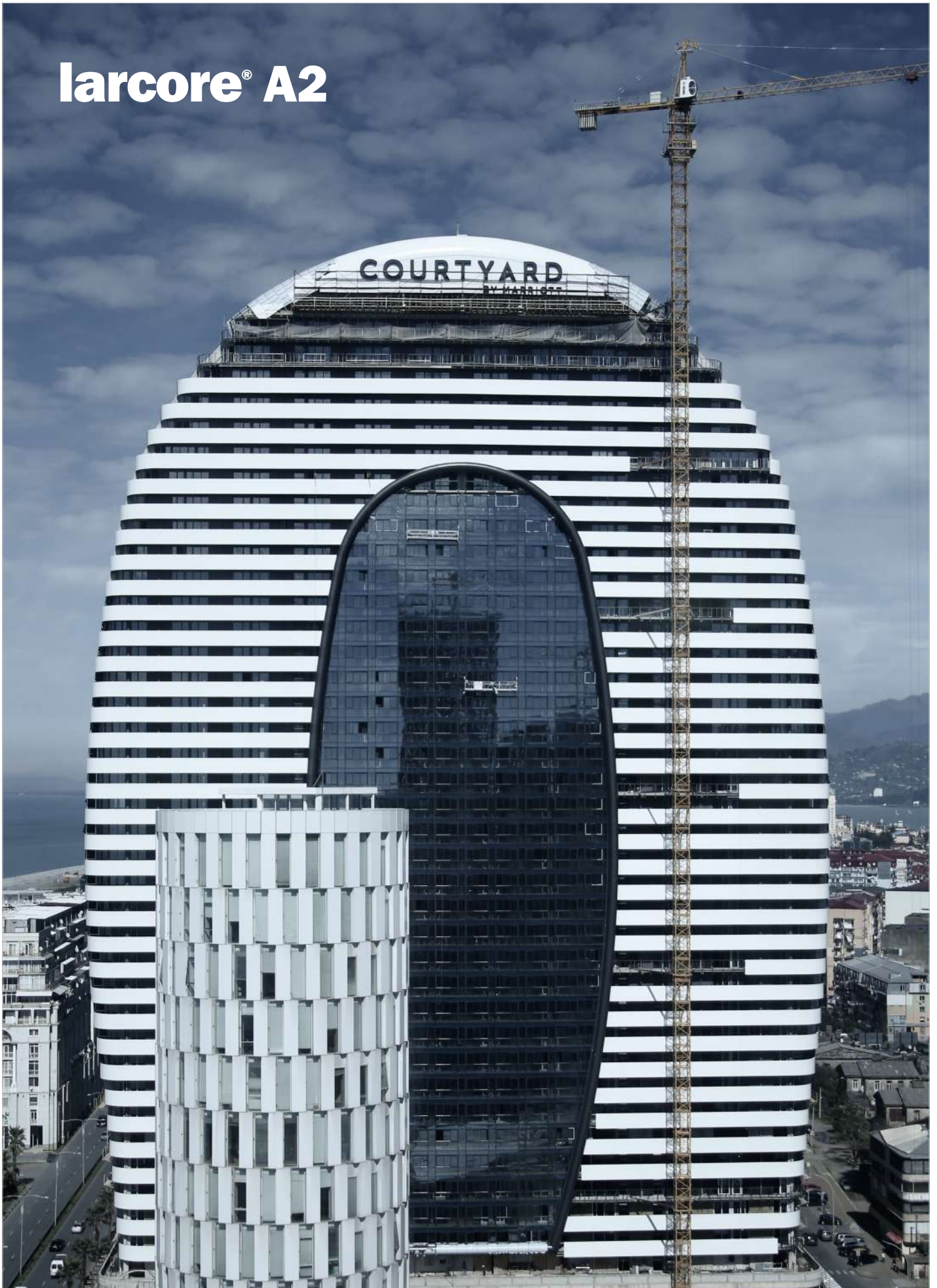
Marriott Courtyard. Batumi, Georgia larcore® A2 10 mm & 8 mm Traffic white 9016 Architects: Alliance Group
